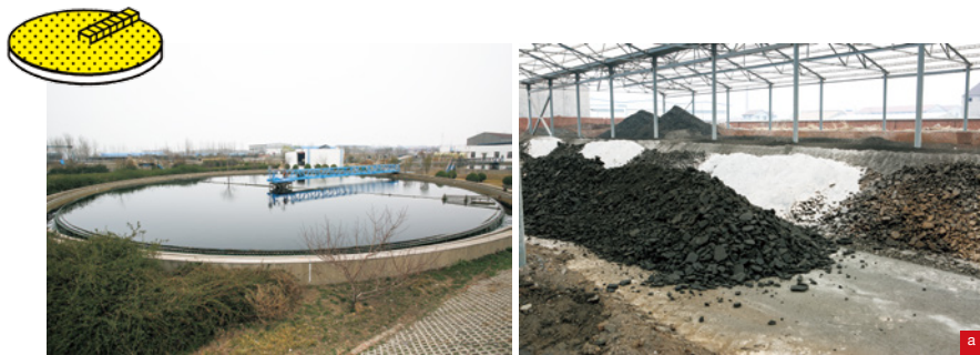
Waste Water Plant
